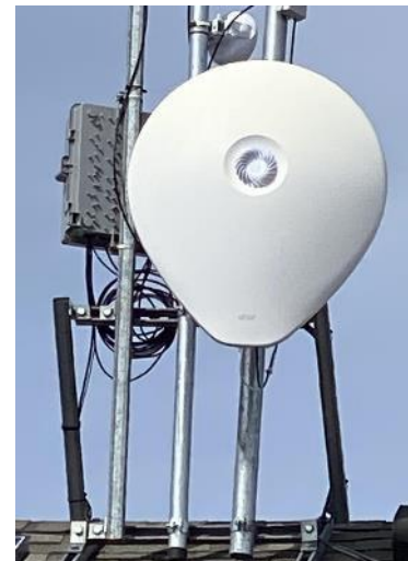
PRM2141 module with 420mm dish and 5GHz backup Approx. > 20 km
